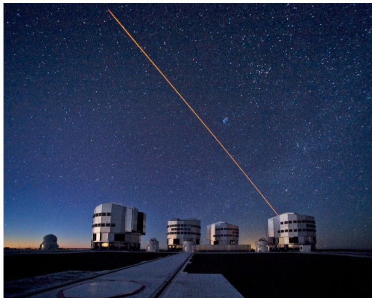
A laser beam projects an artificial guide star into the sky above the European Southern Observatory's VLT facility in Chile's Atacama desert. Adaptive optics systems analyze the beam to cancel out atmospheric turbulence for sharper photos. See this and other photos at the ESO website .
