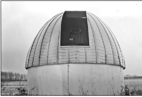
The original dome of the observatory at Rudy Zarling's rural home in Kirchhayn, Washington County in 1974. It was built by Germantown High School students from silo parts. It was vulnerable to high winds and was ultimately destroyed.
