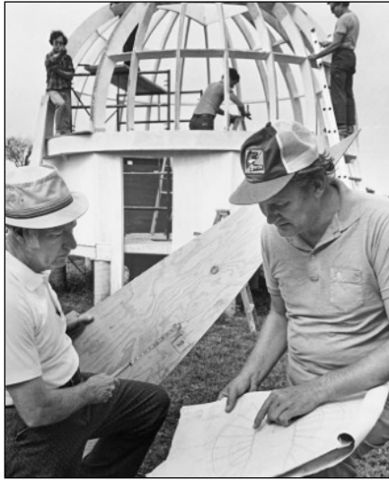
Left: The new dome was built at Carlson Tool and then moved to Zarling's property in 1980, in a project headed by then-president Carl Edquist and Rudy Zarling.
